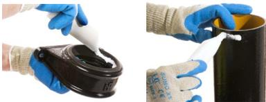
**2)** Apply a small amount of lubricant (TX0001) to the rubber gaskets at both ends of the push fit socket. This is necessary to ensure the insertion of pipes and fittings into the socket.
